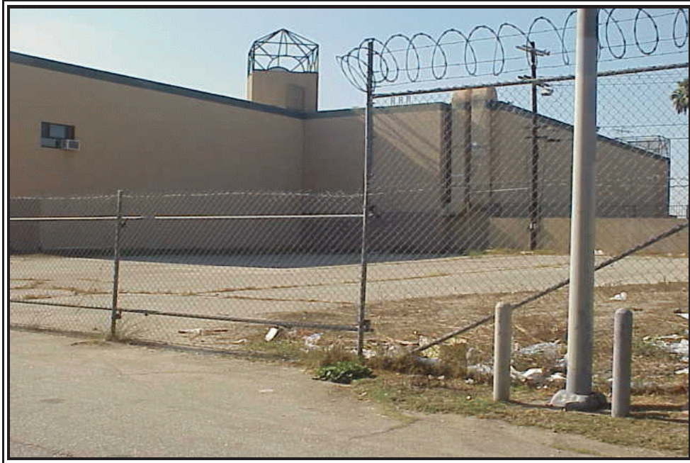
View looking southwest from the northeast corner
